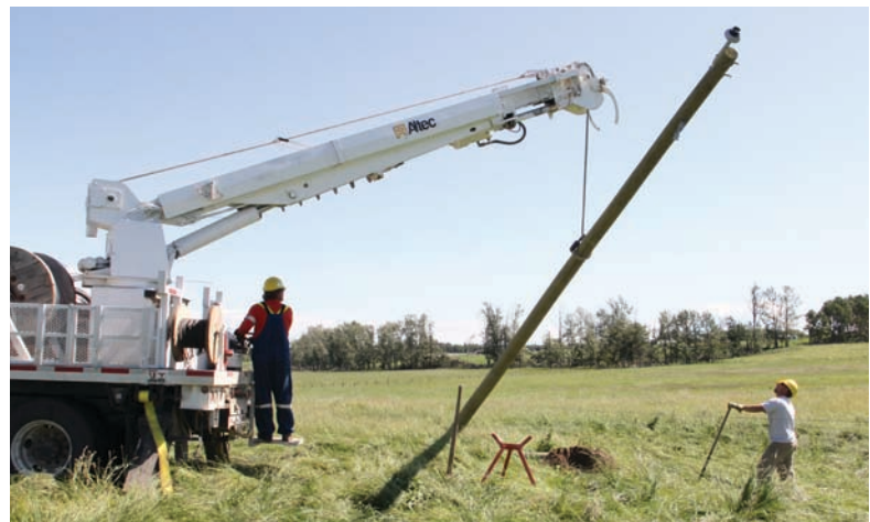
Above, left photo: A barn on Monica Kaban and Mike Burlein's property is missing many shingles and the fencing around it is destroyed. The metal pictured came from the roof of Monica's riding arena. Above, right photo: CAREA Power Line Technicians work to replace a damaged pole along Range Road 21, outside Innisfail, on Thursday, July 7, after a tornado touched down.
