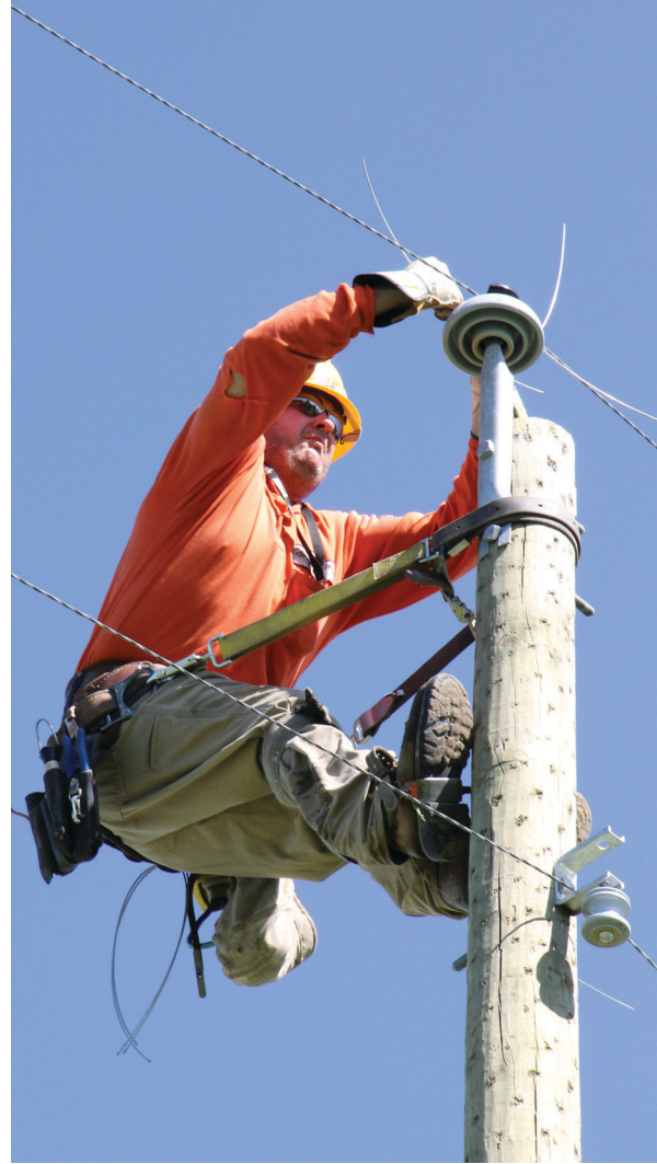
Above photo: CAREA Power Line Technician Darcy Wood climbs a newly-installed power pole to string the power line back up and get the power working again. Left photo: A portion of the metal roof from Monica Kaban's riding arena is pictured laying in her yard.
